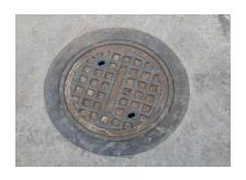
Man holes are located in the front or back yards, they also act like a Junction box where multiply pipe come into these manholes
